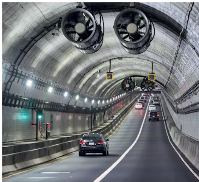
Divestment, Elizabeth River Crossings, Virginia, USA
