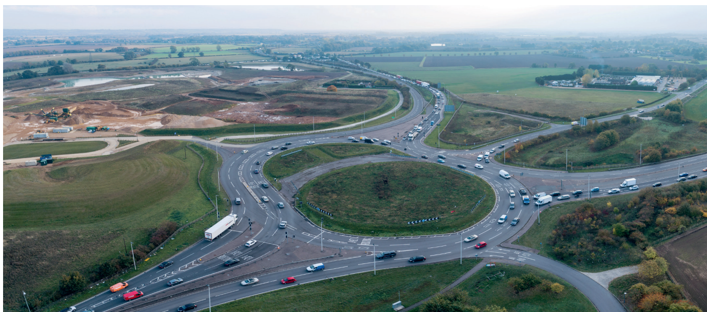
A428 road, East of England region, UK
