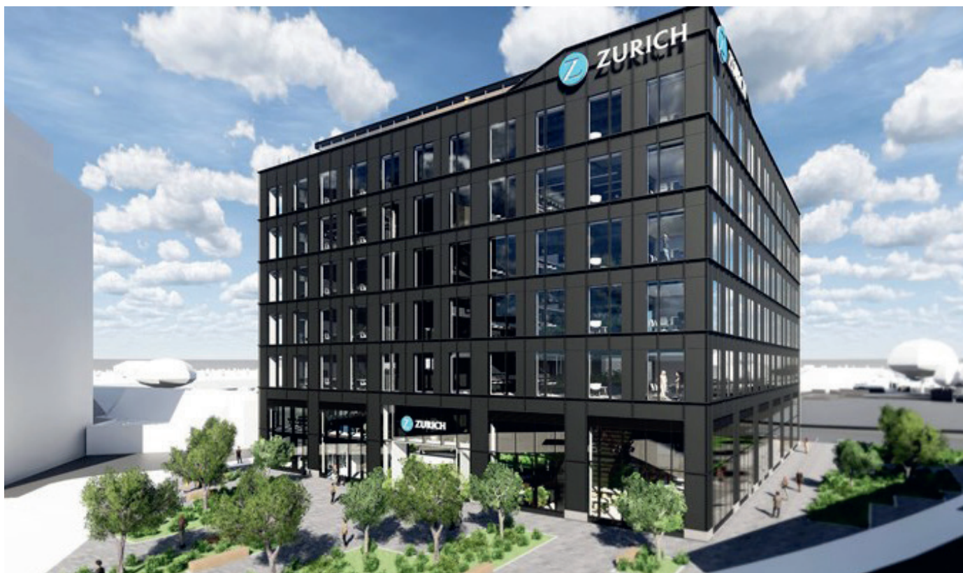
Commercial office building, Swindon, UK
