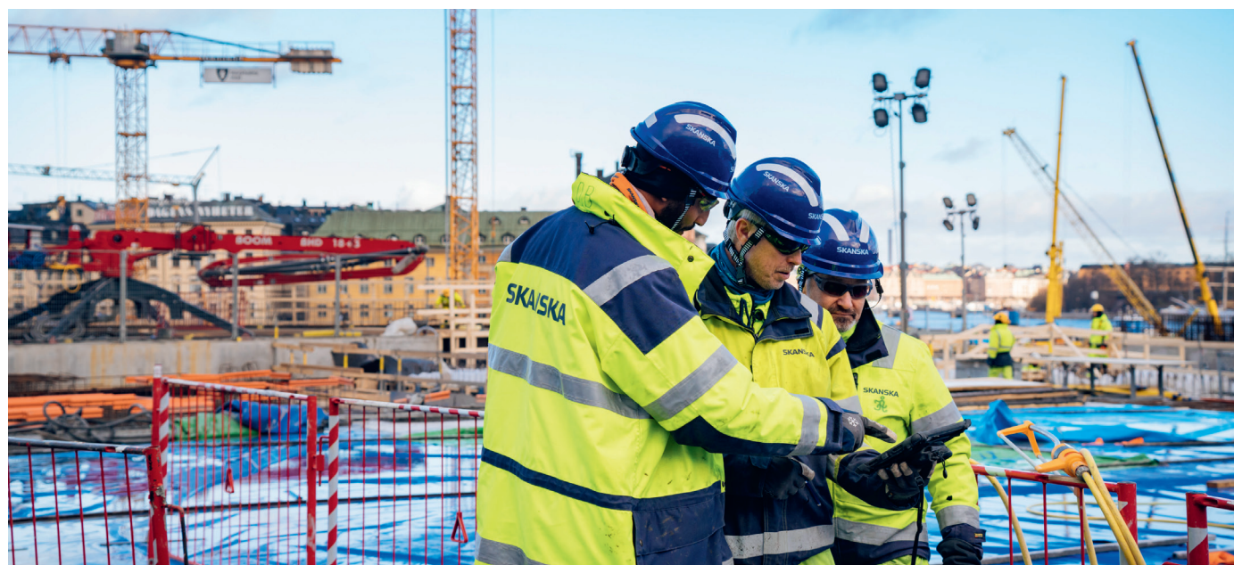
Digital tools on site, Slussen, Stockholm, Sweden
