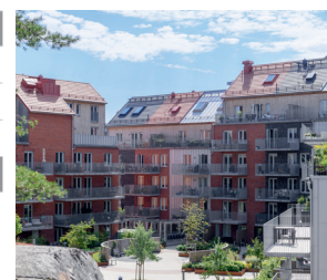
Brf Fritiden, Gothenburg, Sweden
