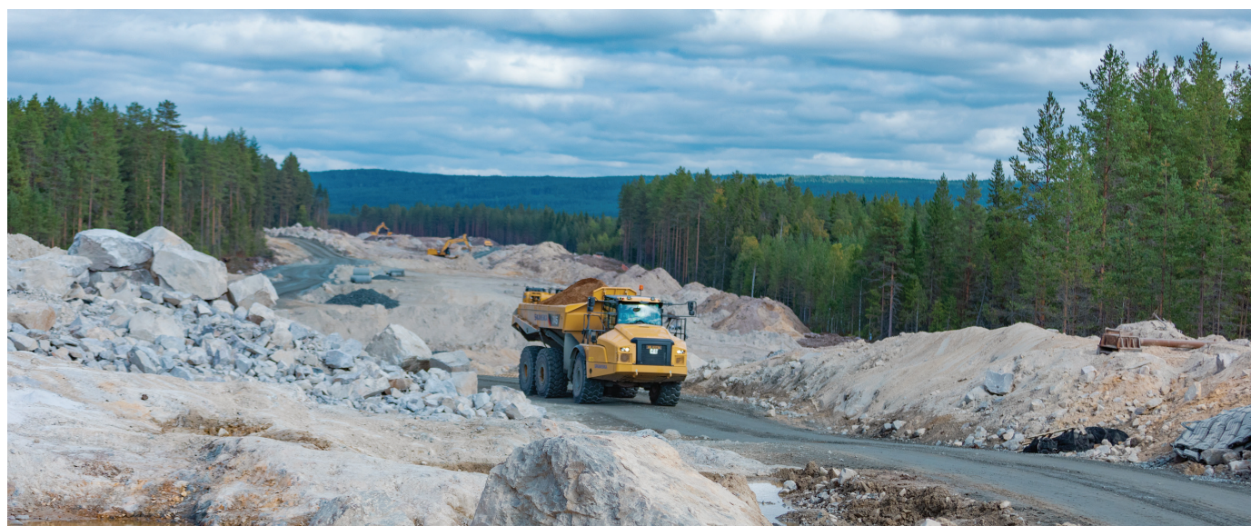
Rv3, road project, Løten to Elverum, Norway.
