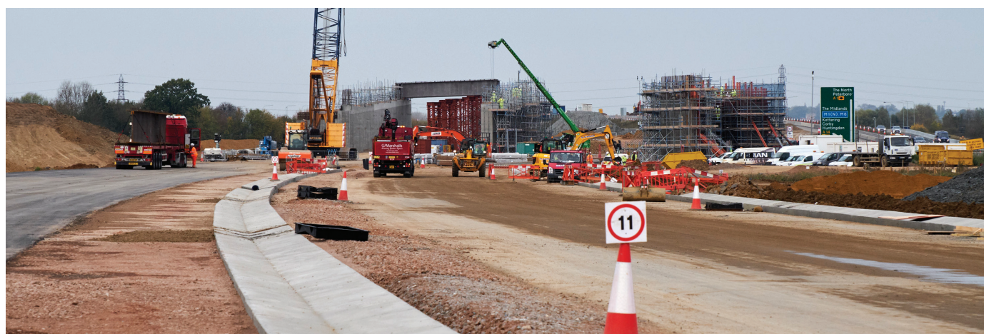
A14, highway project, Cambridge to Huntingdon, UK.
