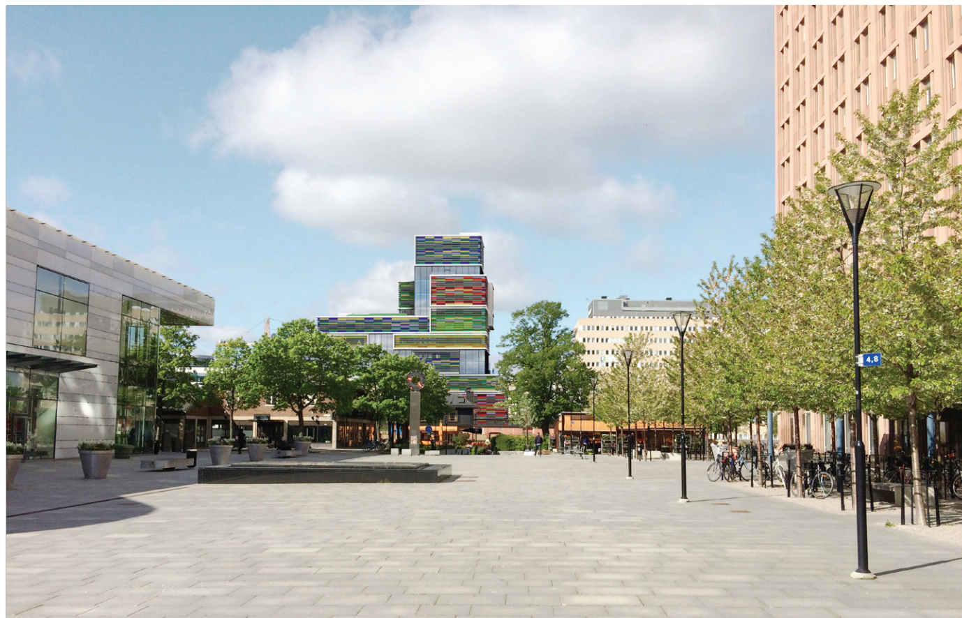
Court- and office building, Sollentuna, Sweden.
