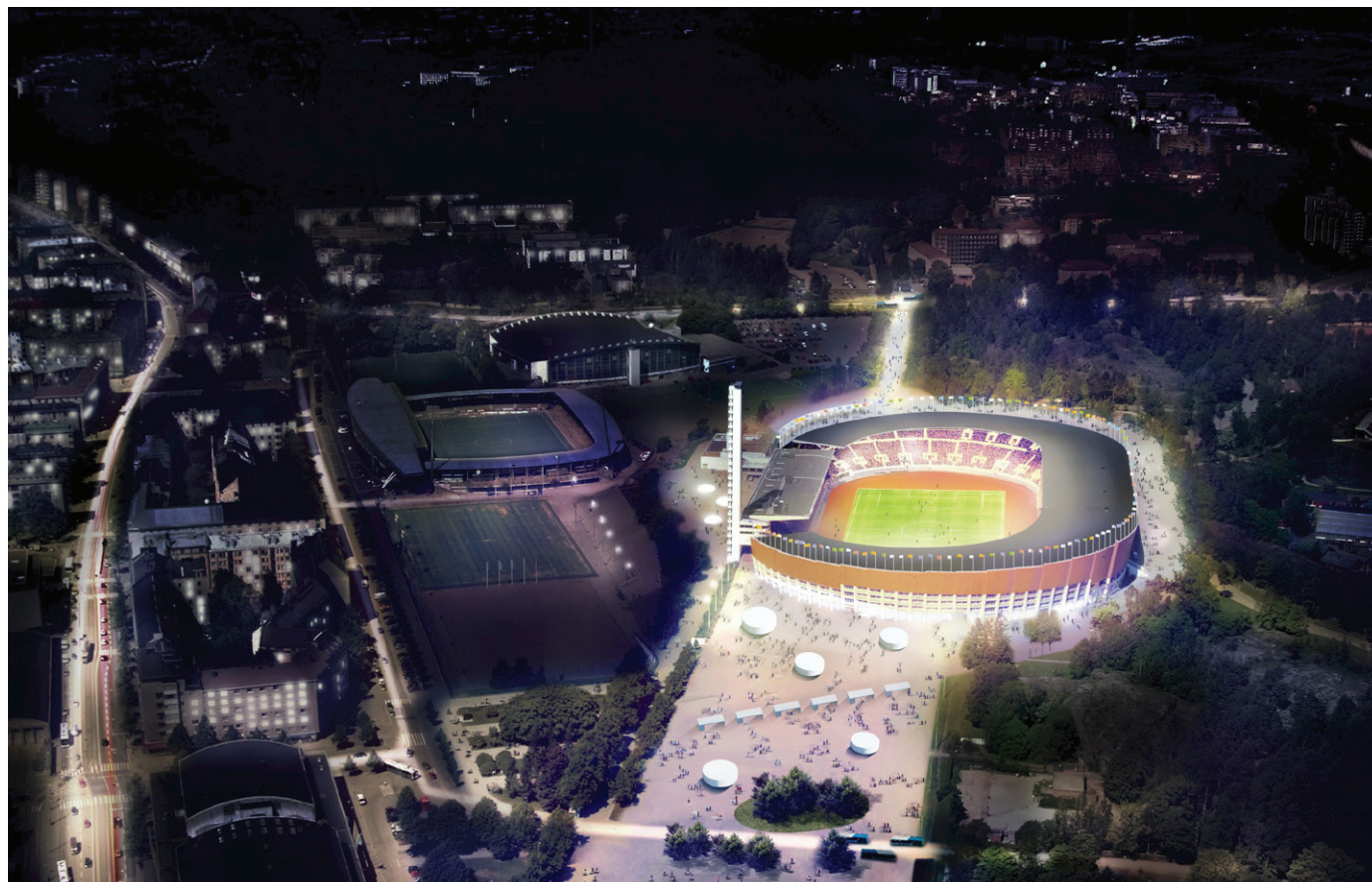
Olympic Stadium, Helsinki, Finland.
