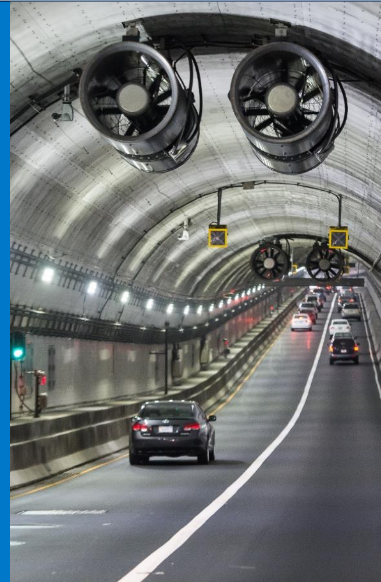
Elizabeth River Tunnels, Virginia, USA
